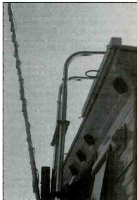
The performance of this high frequency whip improved when it was angled back away from the command post's metal ladder.
